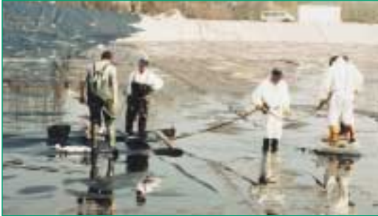
Figure 21 Welding of Carbofol® geomembranes over Combigrd® (tar pond "Neue Sorge", Germany).
