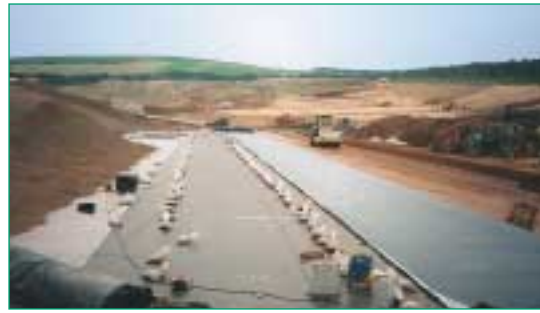
Figure 4 Secutex® protection layer over the HDPE geomembrane (landfill in Germany).
