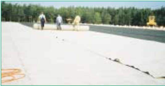
Figure 11 Installation of the Secutex® protection layer (landfill Nurem- berg, Germany).
