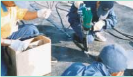
Figure 1 Welding of Carbofol® geomembranes (land- fill Xingfeng, China).
