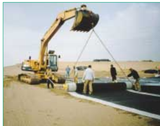
1995, landfill caps were sealed with Carbofol® geomembranes and Bentofix® geosynthetic clay liners.
