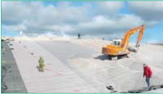
Figure 13 Secugrid® reinforcement above Carbofol® geomembrane and Secutex® protection layer (landfill Ällässlo, Finland).
