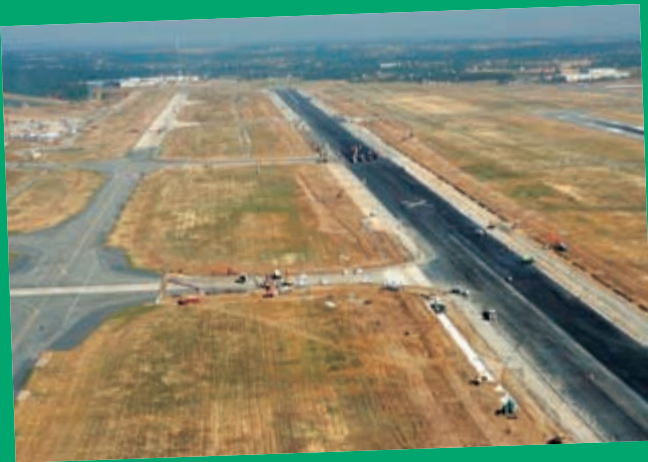
Fig. 1 Runway widening with Bentofix® for environmental protection
