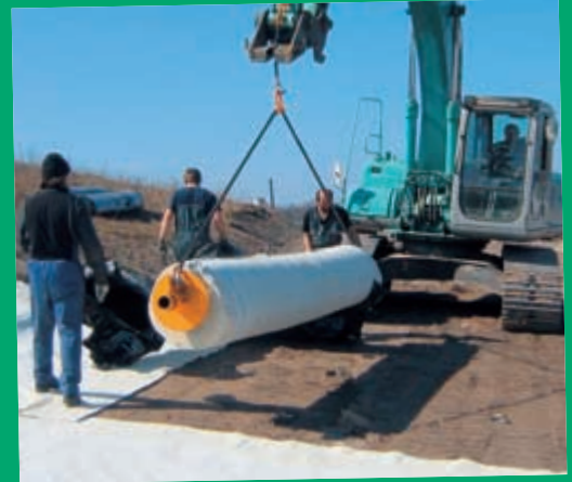
Fig. 2 Bentofix® capping installation
