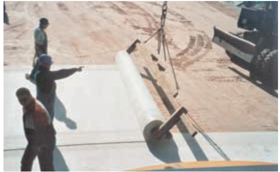
Bentofix® installation
