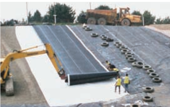
Geomembrane installation over GCL
