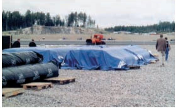
Storage on site
