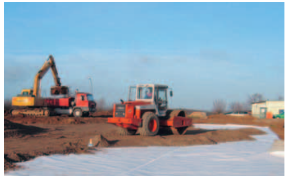
Soil compaction over Combigrig®
