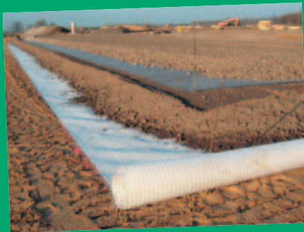
Fig. 4 Combigrid® installation over the soft subgrade (Kuestrin-Kietz, Germany)
