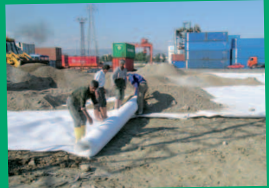
Fig. 5 Unrolling and overlapping of Combigrid® over the soft subgrade
