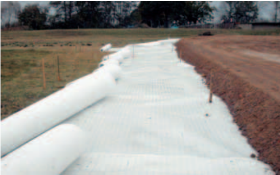
Installed Combigrig® with overlaps
