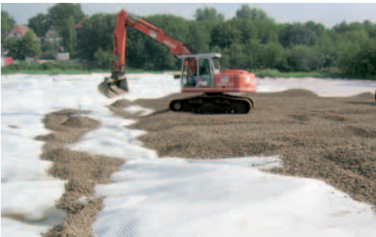
Placement of min. 200 mm aggregate
