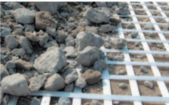
Interlocking of soil aggregate
