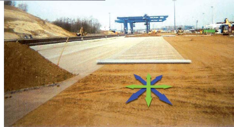
Figure 4 Potential stress directions in geogrid reinforcement layers
