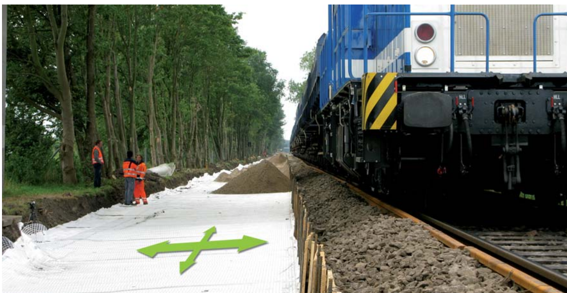
Figure 4 Potential stress directions in geogrid reinforcement layers
